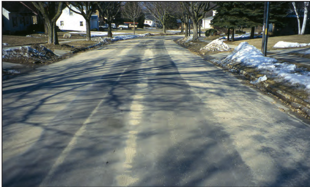
Figure 19. Residue from sand applied to a street surface to provide traction for vehicles.
